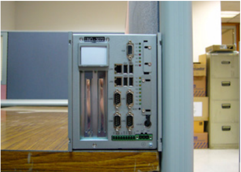
Figure 3.6: UNO-3072 Improper Installation (2)
