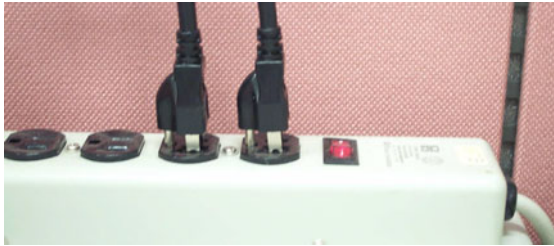
Figure 3.9: Power cord plugs orientation on the socket
